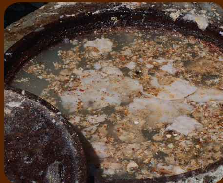
Neglected Grease Trap
