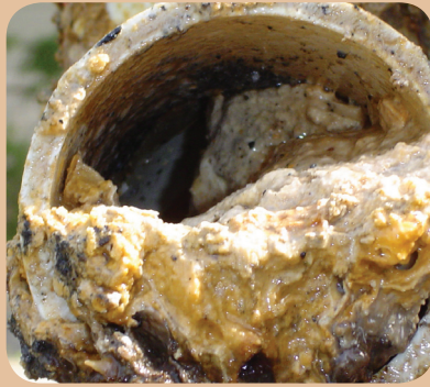
FOG in Sewer Line
